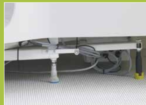
Electronic box sits neatly into metal brackets under bath for access. Magnets plinth brackets
